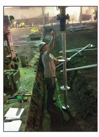
The (16) 2.875" diameter helical piles manufactured by IDEAL Group were installed to an average depth of 24 ft. to a capacity of 34 kips ultimate capacity. After the piles were cut to the specified elevation, 8" x 8" plate caps were installed on the top of the piles prior to the installation of the rebar. All of the helical pile installation work was completed in (1) day.
