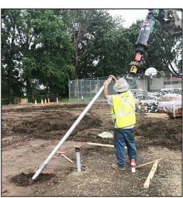
Hunter Modular Construction contacted SSRG to help develop a helical pile foundation solution for the modular building complexes for Little Ferry Board of Education. After a few engineering discussions and reviews, the structural engineer designed (212) helical piles acting as a foundation for two building complexes.
