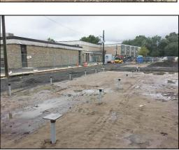
During installation of piles, the crew had challenges working in heavy rains for a couple of days. However, the rains did not stall the work schedule thus affirming the use of helical piles as a better solution in adverse weather conditions.
