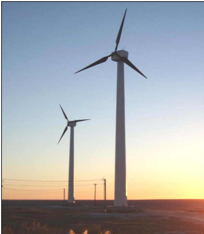
Fig. 5. Operational Northwind 100 wind turbines at Kasigluk.
