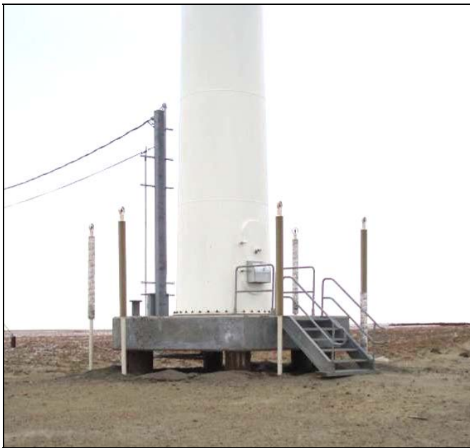
Fig. 4. Kasigluk wind turbine foundation completed, including power drop and thermosyphons.
