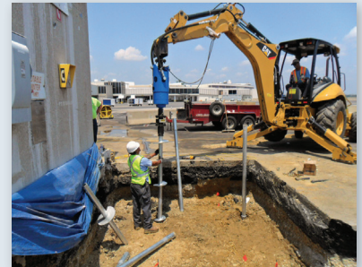
Aligning drive head and pile for installation
