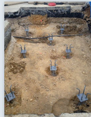
Pile installation complete
