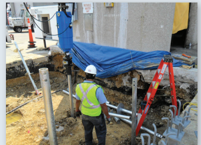
Advancing helical pile
