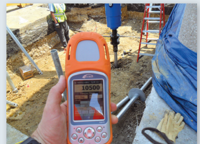
Monitoring torque during installation
