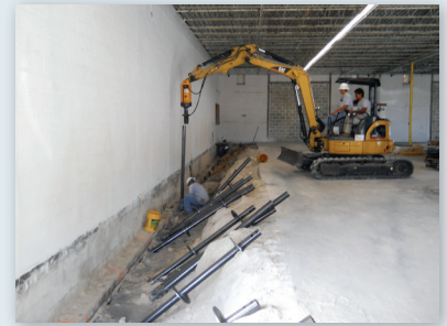
Vertical piers installed inside warehouse
