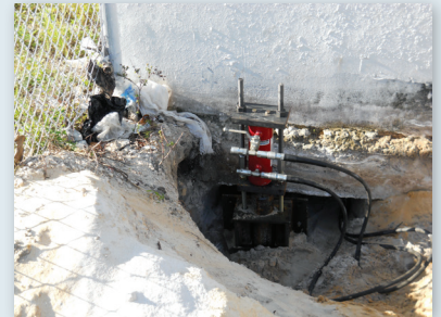
Hydraulic cylinders preload piers before excavation
