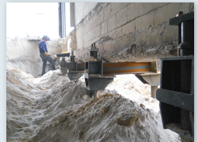
Steel beams welded to retrofit brackets
