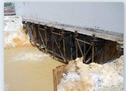
Excavation of contaminated soil. Building stabilized with helical piers.
