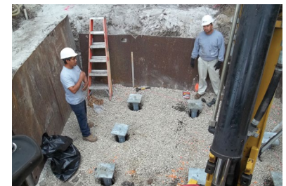
Helical piles fitted with new construction brackets
