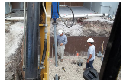
Installing helical piles
