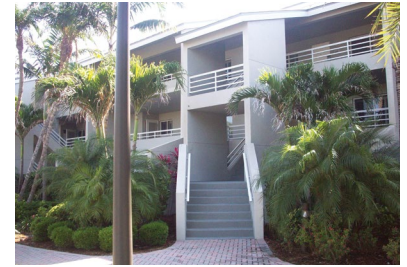
Proposed location for new elevator addition
