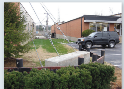
Finished grade beam reaction system at the northwest guy location
