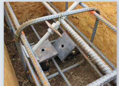
Concrete grade beam reinforcement
