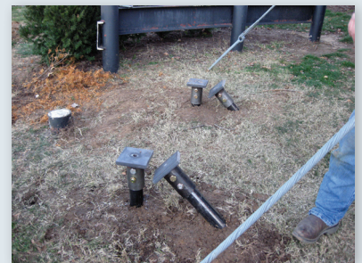
Compression and tension pile system installed at the northwest guy location
