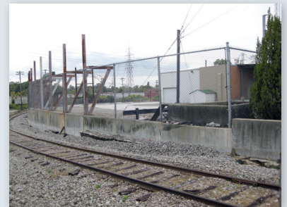
Northeast guy pole and adjacent railroad easement; prior to retrofitting
