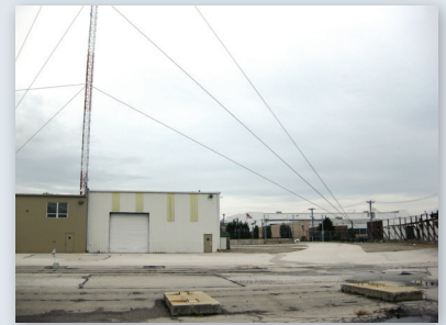
Tower with northeast guy pole on right
