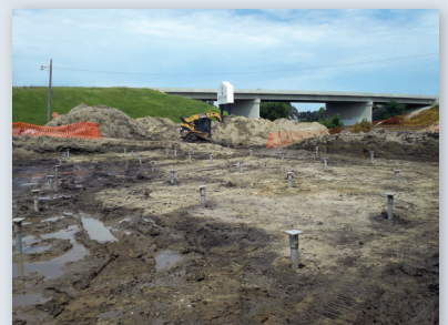
Completed pile installation
