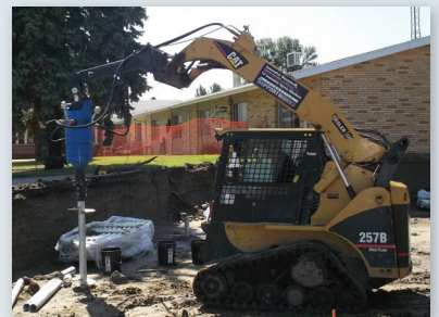
Piles installed with tracked skid-steer
