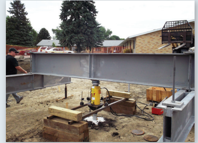
Load frame centered over helical pile
