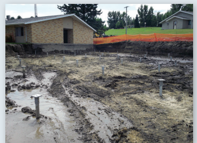
Completed pile installation
