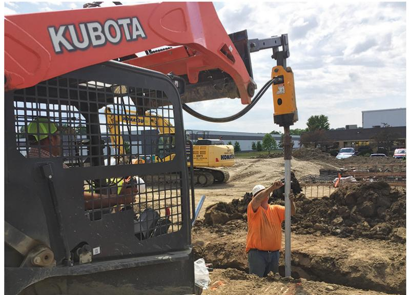
Installing ECP Helical Screw Piling
