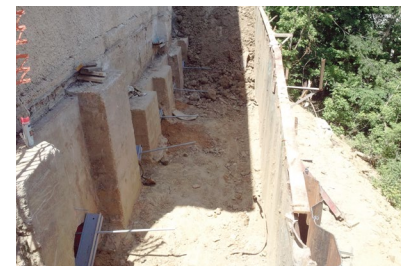
Tiebacks advanced through core holes of concrete underpinning
