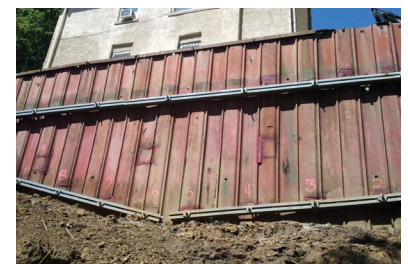
Tieback and waler installation complete
