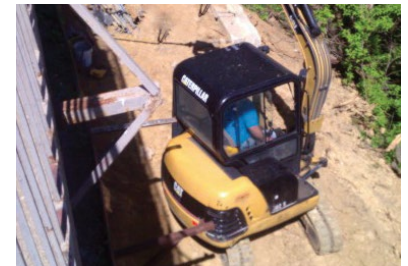
Maneuvering for tieback installation
