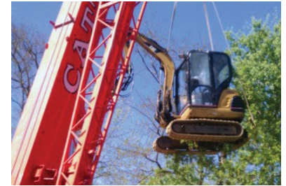
Lowering mini-excavator onto working surface below wall
