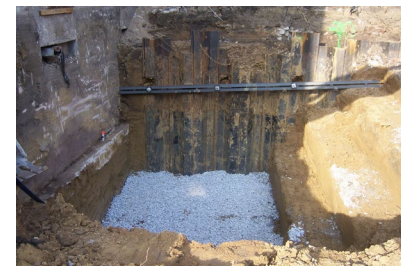
Tieback and waler installation complete
