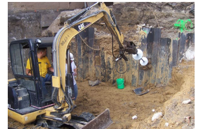
Tieback lead section advanced through sheet pile wall
