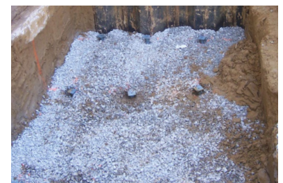
Completed pile installation
