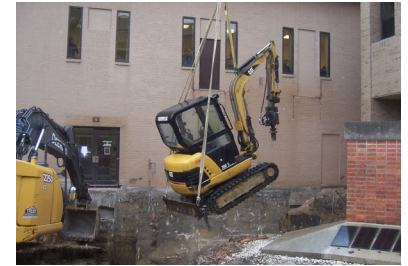
Lowering mini-excavator into excavation
