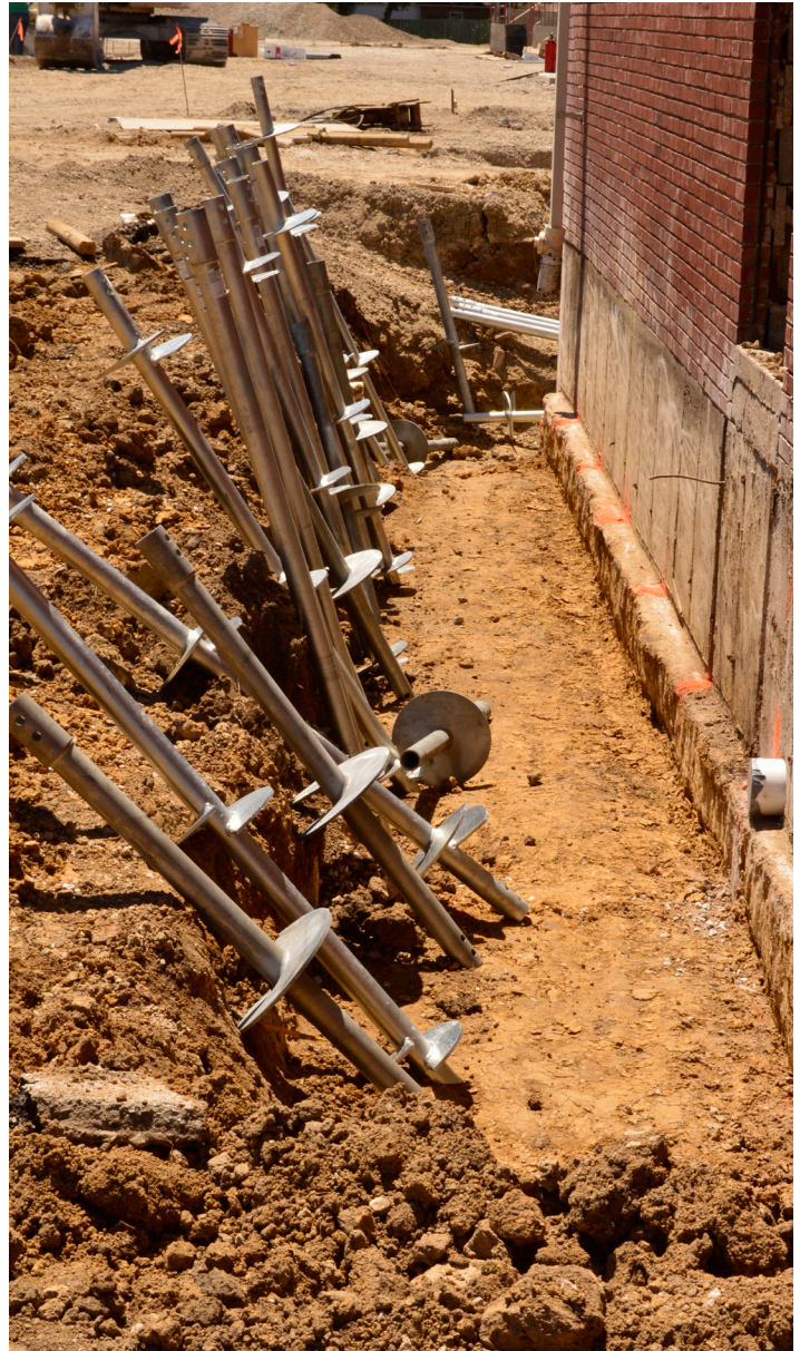
Product staged along east gym wall; looking south
