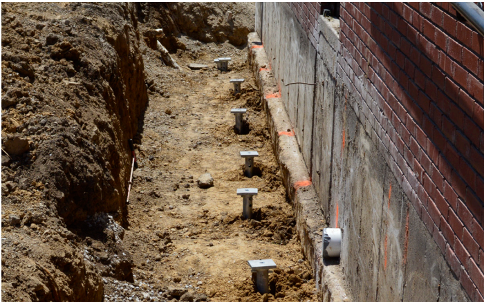
Pile installation complete
