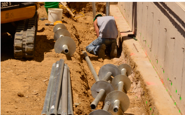
Helical pile installation along south wall of gym
