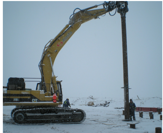
Figure 2. Typical helical pile installation
