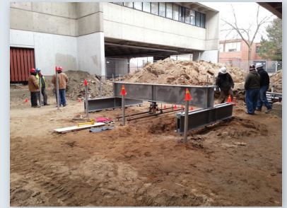
Compression field load testing prior to installation of production piles
