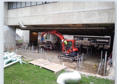
Area of limited headroom; vertical and battered piles installed
