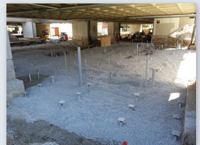
New construction pile caps field welded in place
