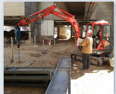
Advancing helical pile lead section
