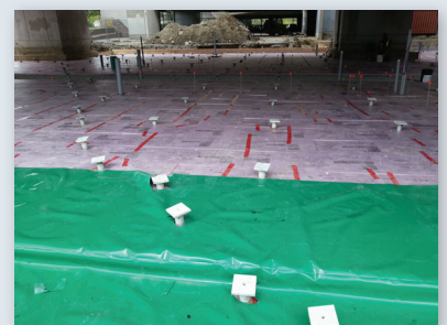
Methane gas barrier system being installed around helical piles
