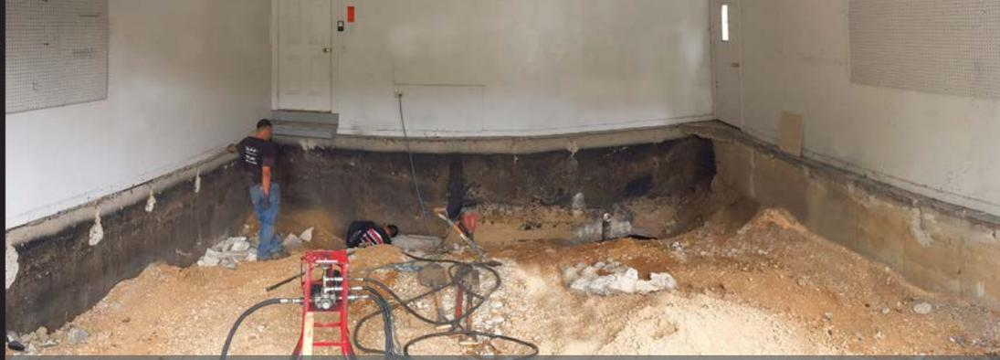
Installation of helical piles to remedy sinkhole damage to basement
