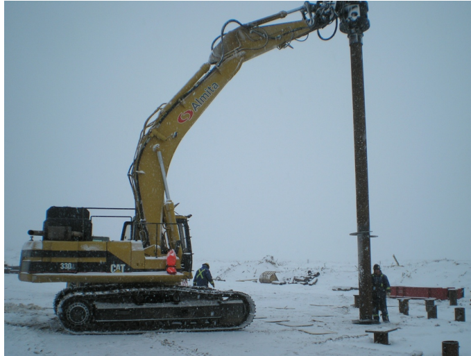
Fig. 2. Typical helical pile installation
