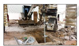
In addition to the (21) helical piles with underpinning brackets, (2) additional helical piles were installed with concrete pile caps to support the front concrete stair case walls. The new foundation has a height of (8) feet, and the walls are (8) inches thick with (2) #5 rebar horizontally on the top and bottom and vertically (3) feet on center. (11) Smart Flood Foundation Vents were installed to alleviate future hydrostatic water pressures.
