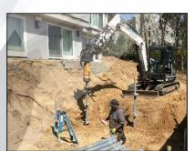
(35) Chance 2.875" diameter round shaft helical piles were installed to an average depth of 26 feet to support the walls and grade beams.
