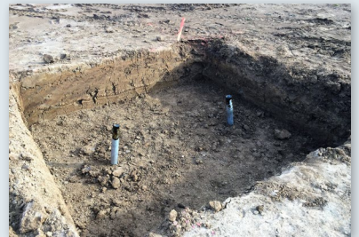
Helical piles installed to specified elevation
