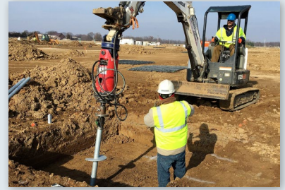
Installing battered lead section
