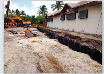
Sheet pile wall installed behind parking garage
