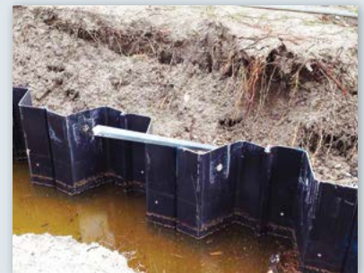
Tieback installed, ready to be cut and fitted with standard new construction bracket
