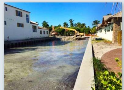
Seawall caps poured and inlet dredged
