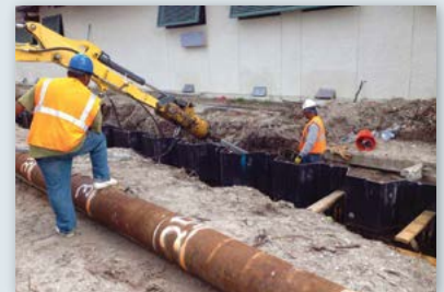
Advancing tiebacks from top of sheet pile wall
