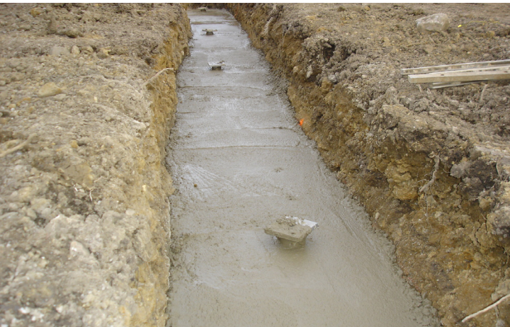
Concrete "mud mat" poured to receive wall
