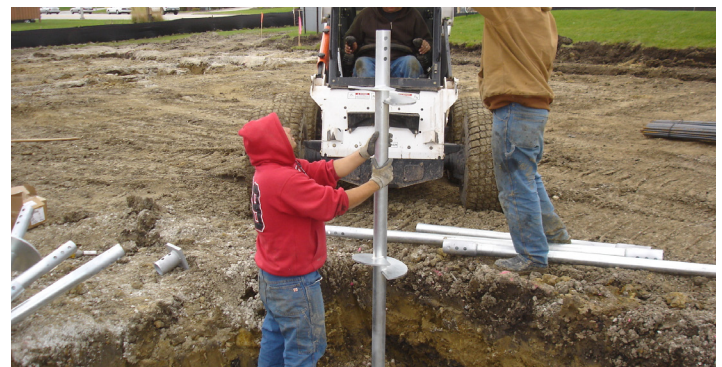
Lead sections advanced
