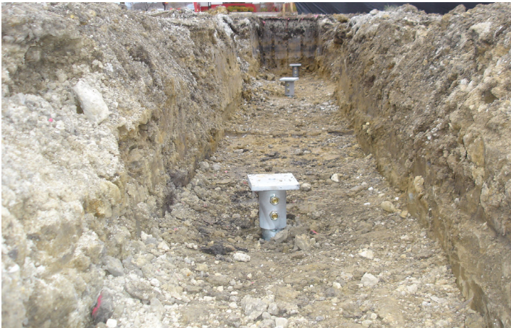
Pile caps installed
