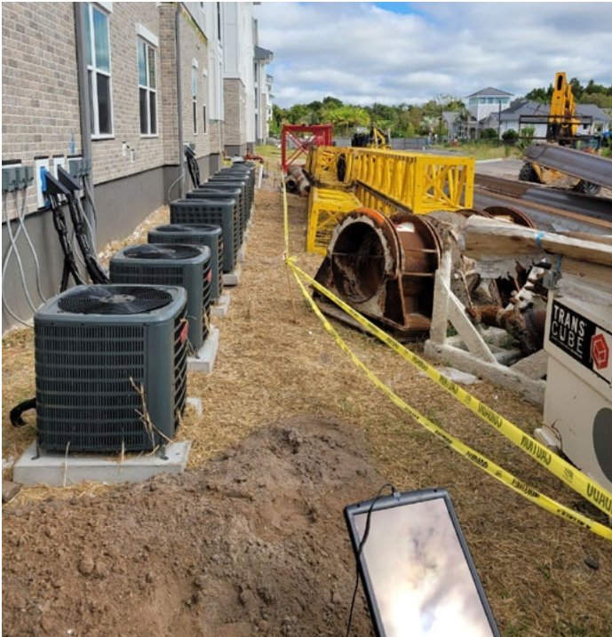
East wall of Aventon Lana housing complex prior to removal of AC units
