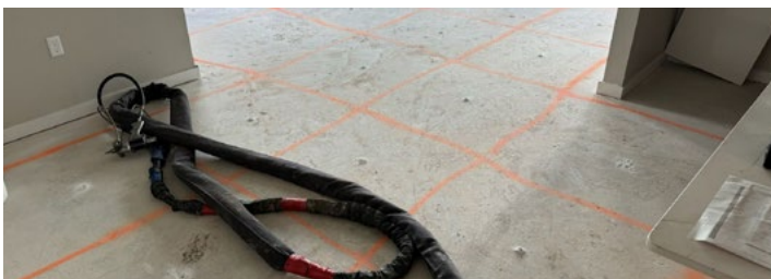
Polyurethane foam injection at interior slabs
