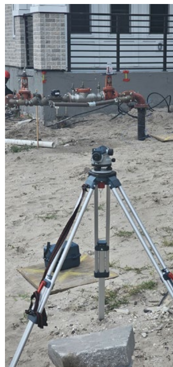
Monitoring structural lift with survey instruments
