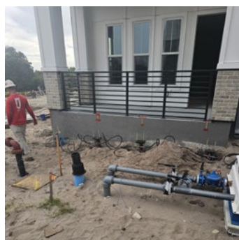
Retrofit brackets with lift cylinders attached
