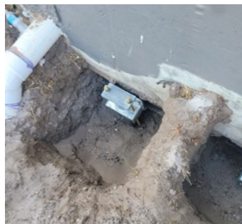
Retrofit brackets installed
