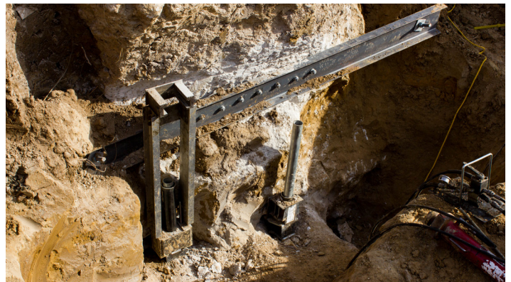
Tiebacks and waler installed; Retrofit brackets positioned for push pier installation
