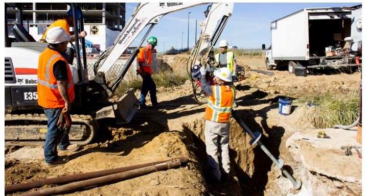
Positioning helical tieback lead section for advancement
