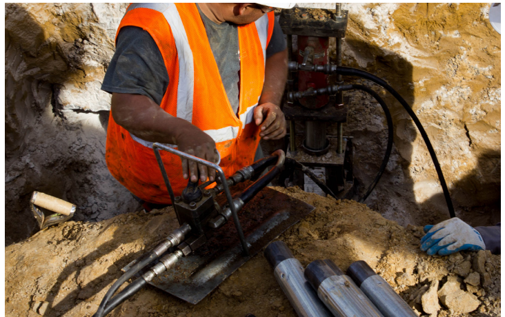
Reloading push pier to design working load
