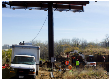
Billboard and adjacent retaining wall construction
