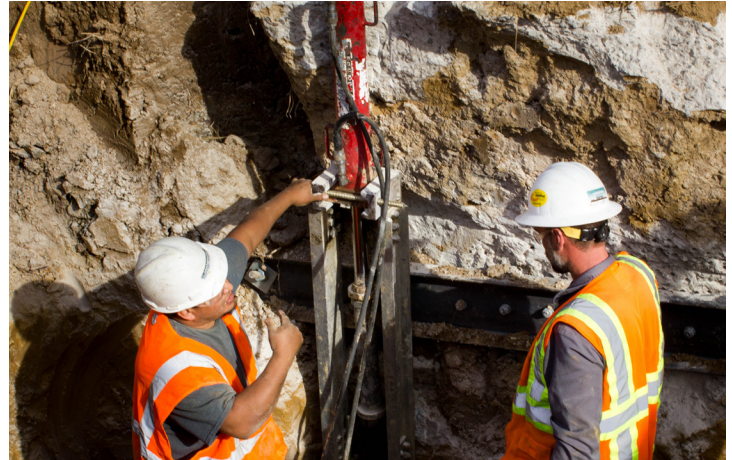
Driving PP288 push pier
