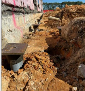
Installed & Cut at Design Installation
