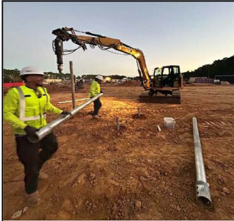
Installing Test Pile & Four Reaction Piles
