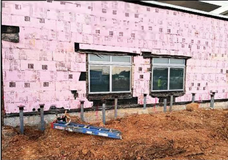
Several Piles Installed
