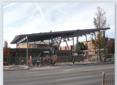
Proposed addition under construction
