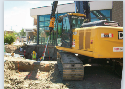
Track excavator installing battered HP450 helical piles
