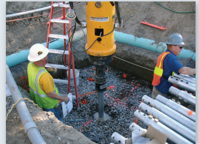
45 kip-ft drive head installing helical piles
