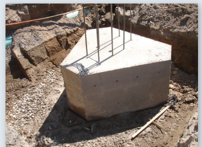
Helical piles cast into concrete pile caps
