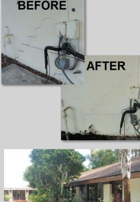
**Situation:** The Chick-Fil-A lodge overlooking the Sugar Mill Golf Course in New Smyrna Beach, FL was experiencing signs of foundation settlement. There were stair-step cracks and wall separation along the entire exterior of the building facing the lake. The property management company reached out to Ram Jack for a minimally-invasive solution to their settlement problem.
