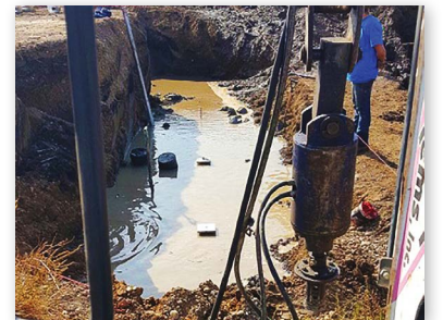
Piles installed through standing water
