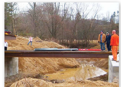
Abutments poured and bridge decking placed
