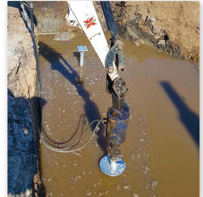
Installing lead section from above excavation
