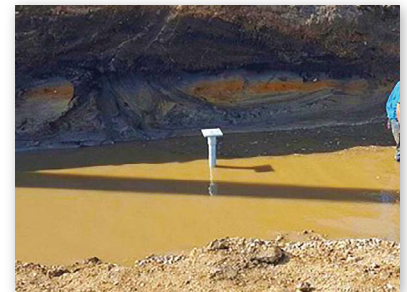
Pile installed to specified elevation
