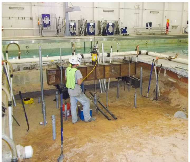
Tension load test
