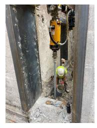
made of steel, was placed just below the coupler. This allowed the grouted columns to continue to a load bearing stratum target depth of 30-35 feet. After reaching the target depth, the concrete piles were capped with new construction pile caps with number 6 rebar full cages.
