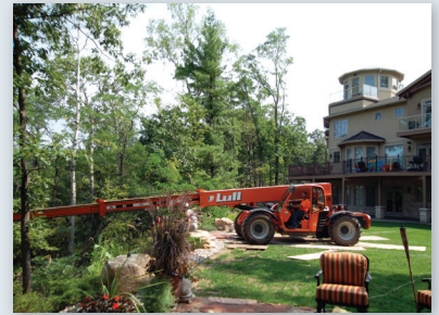
Installing piles with extended boom of material handler
