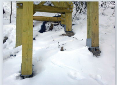
Saddle bracket connection to columns
