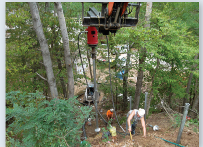
Steep slope; advancing lead section
