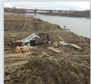
Helical pile installation through levee
