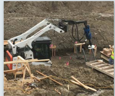
Installing battered piles
