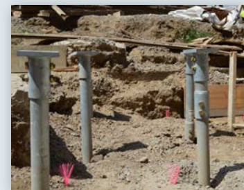
Installed piles
