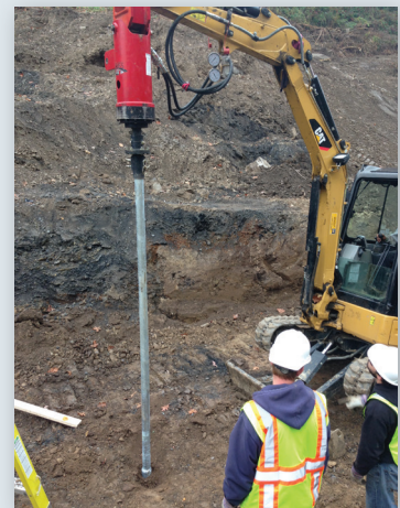
Installing helical pile
