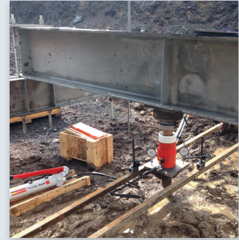
Compression load test
