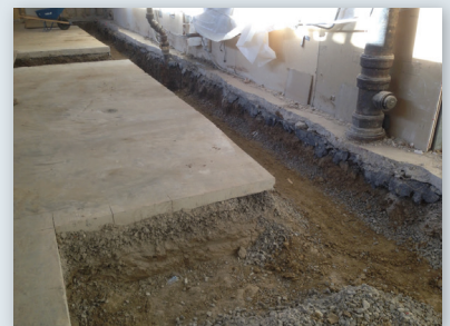
Demolition completed for pile installation
