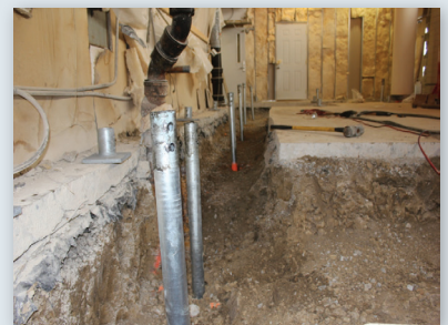
Installed piles to be cut to design elevation
