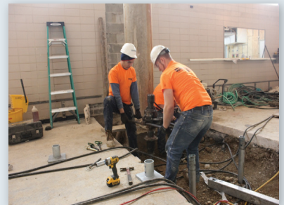
Helical piles installed with hand held equipment
