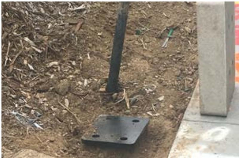
fin collar just below the transfer plate. This will be pulled into the soil by the helical plate to provide lateral stability.
