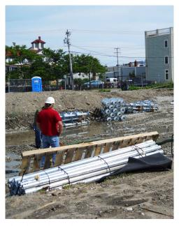
The photo above shows *ECP Torque Anchor*<sup>imestarrow</sup> product on the job site. Above one can see the lead sections with the 12"-12"-14" diameter plates at the center of the photo. Extension sections are at the bottom of the photo. Extensions are used to achieve the specified depth requirement.
