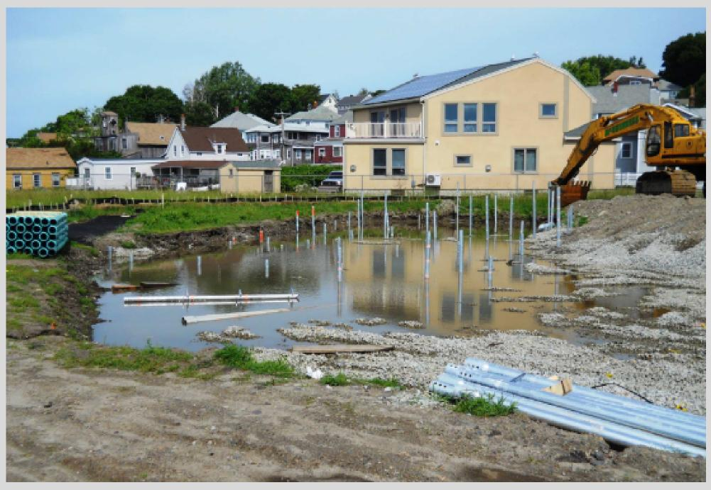
Several major challenges had to be addressed including working during the local tidal changes and with high water table on site. The weak soil also generated concern that the piles may have trouble getting the required torque to adequately support the design loads.
