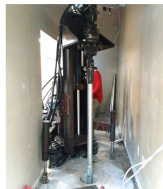
Installing helical slab pier in tight access area
