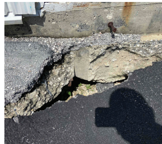
Exterior footing condition prior to underpinning
