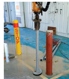
Installing helical slab pier in auction lane area
