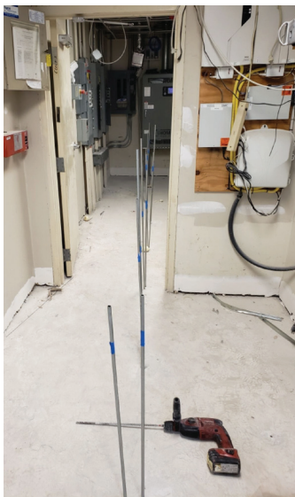
Deep injection tubes for PolyLevel installation at Electrical and IT Rooms
