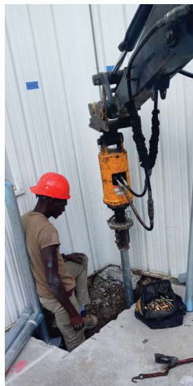
Installing helical pier at exterior footing
