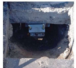
Exterior footing helical pier with underpinning bracket installed
