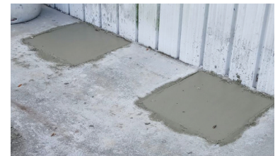
Exterior pier locations backfilled, and concrete finished
