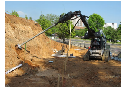
Installation of helical tieback
