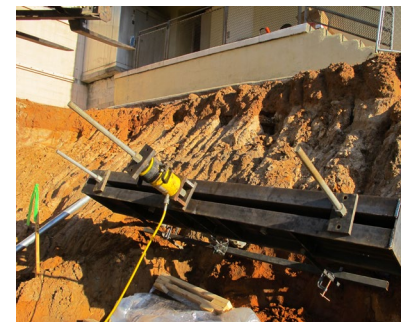
Load test set up (tension)
