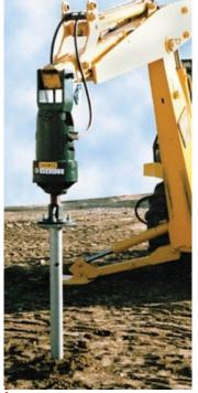
Torque correlation method yields more consistent results than either of the other two methods and is best suited for on-site production control and termination criteria
