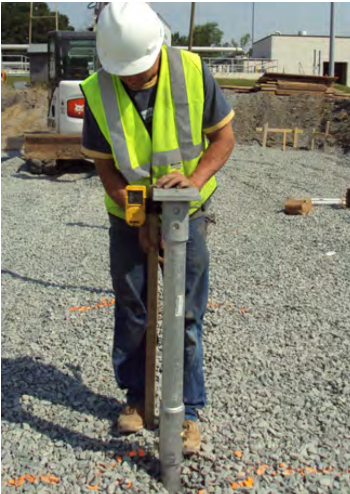
Verifying top of pile elevation
