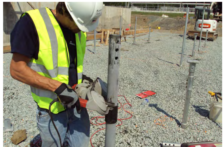
Cutting pile to design elevation with portable band saw
