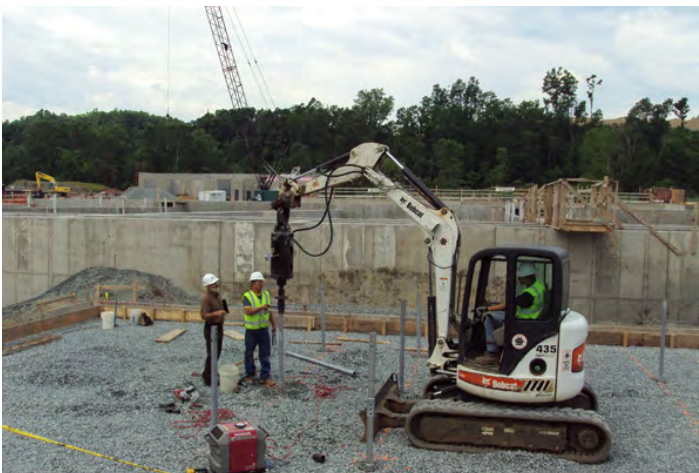
Advancing helical piles
