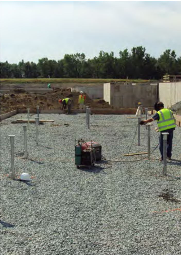
Piles installed, bracket tack-welded
