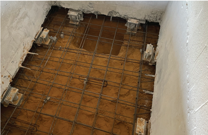
Reinforcement installed in new floor location
