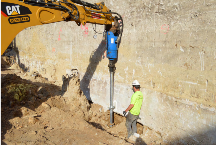
Advancing helical pier lead section
