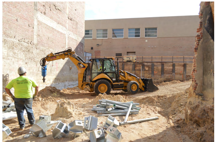
Positioning equipment for helical pier installation
