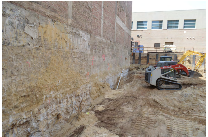
Exposed foundation wall of existing building
