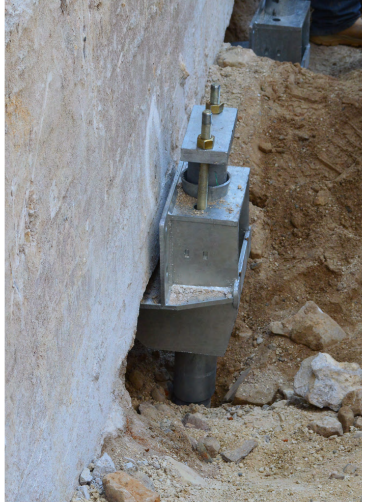
Retrofit bracket installed
