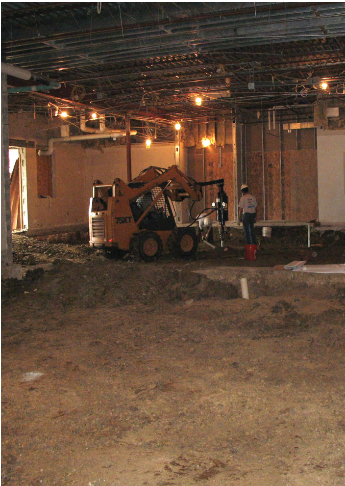
Piles are installed in limited access areas within the building using small construction equipment
