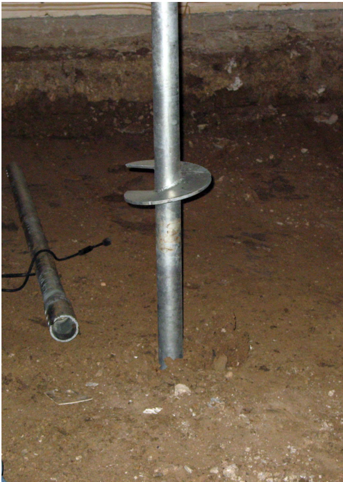
Advancing lead section through hard, dry to damp fill soil
