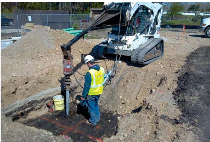
Helical piles advanced at isolated column location
