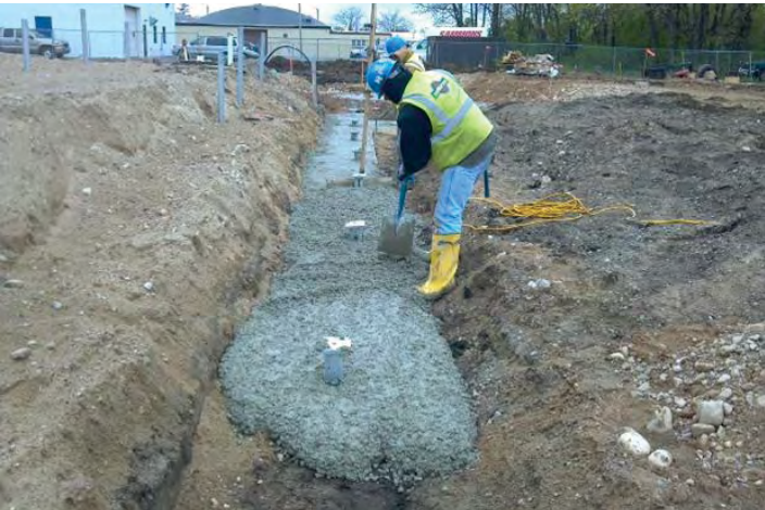
Concrete mud mat placed to support forms for grade beams (foundation walls)
