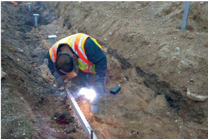
New construction brackets tack-welded to piles
