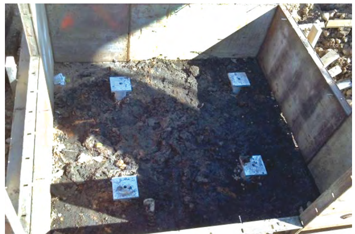
Helical piles installed at column pad
