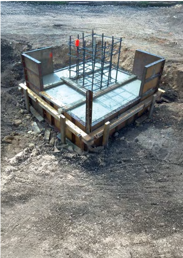
Completed pile-supported column pad
