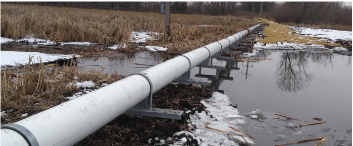
Steel cradle and helical piles support pipeline
