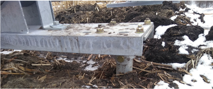
Connection of helical pile to cradle support
