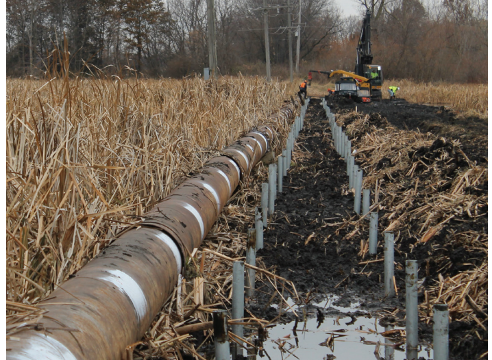
Installing helical piles adjacent to the existing pipeline and overhead utilities
