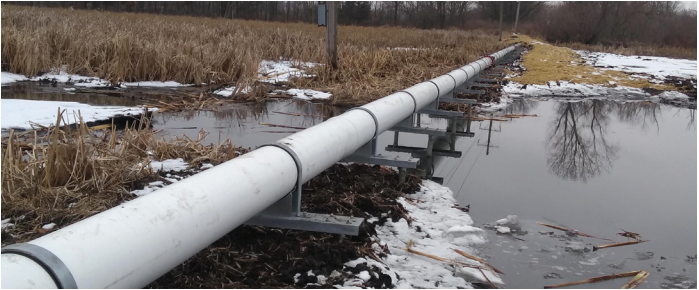
Steel cradle and helical piles support pipeline
