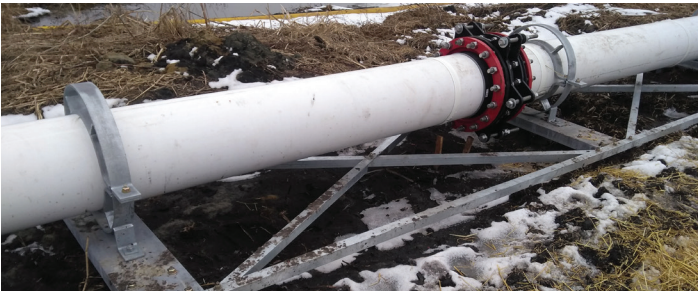
Pipeline support at an expansion joint
