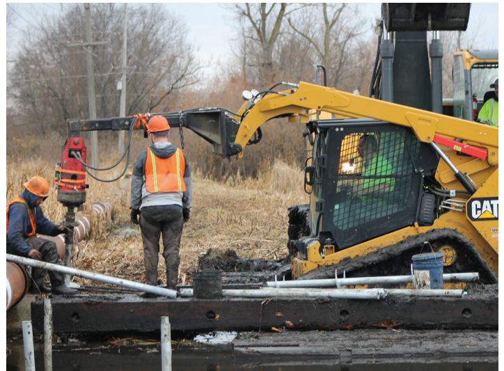
Timber matting support for the pile installation equipment
