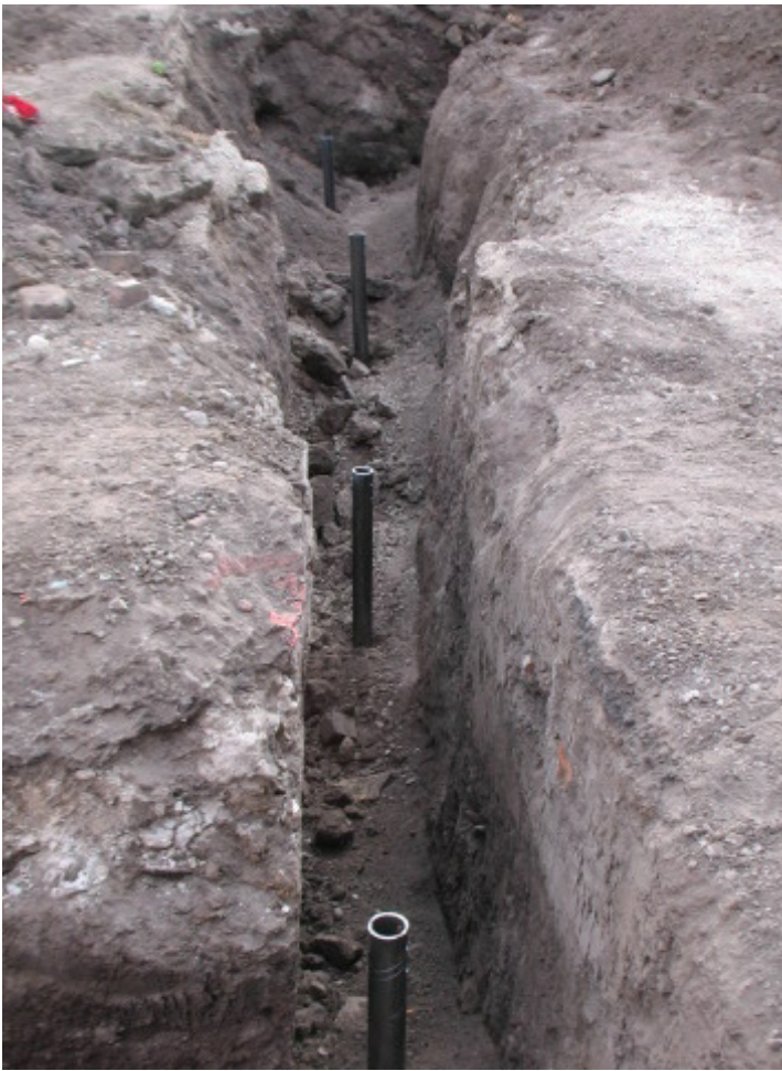
Installed piles in grade beam trench to be cut and fitted with new construction brackets
