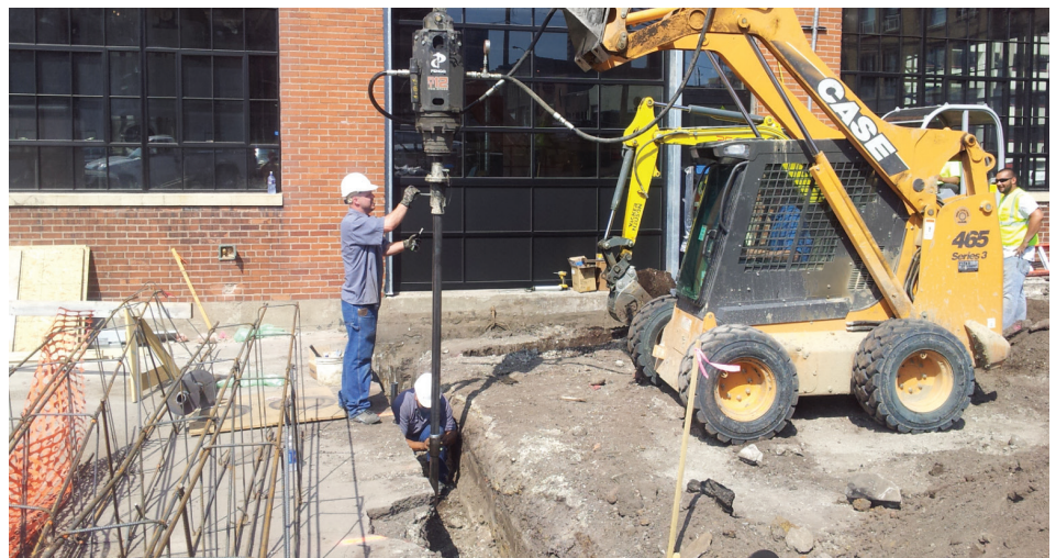
Advancing piles with standard extensions
