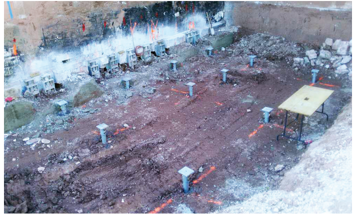
Helical piles installed for addition; push piers installed along existing footing
