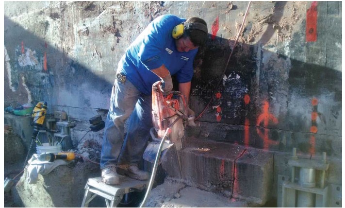
Preparing footing for push pier retrofit brackets
