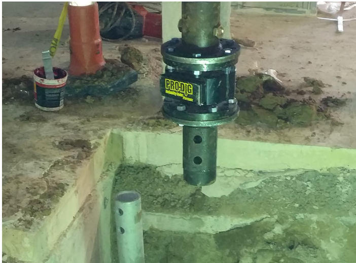
Calibrated torque transducer used to measure and record torque
