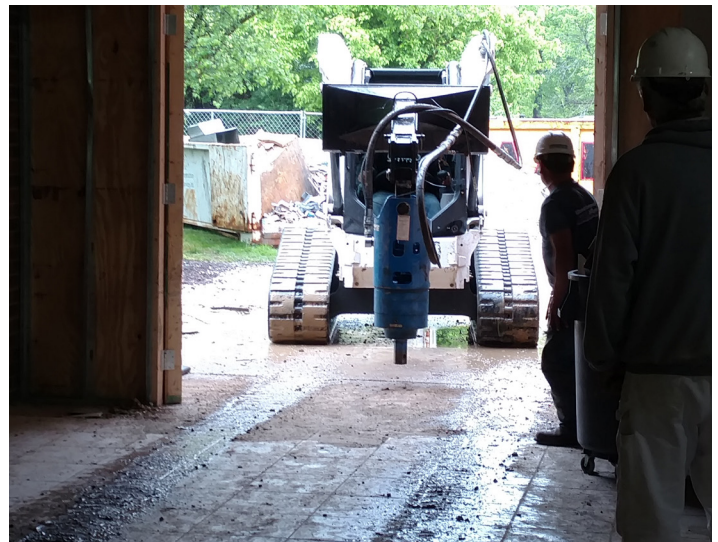
Skid steer with drive head entering building
