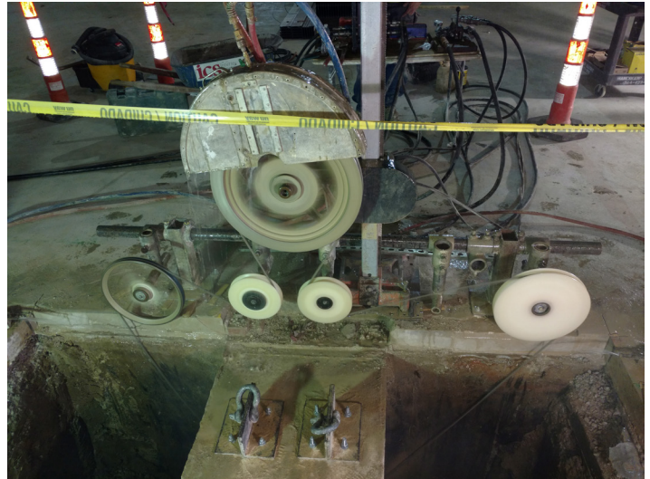
Cutting concrete deadman free from tunnel wall
